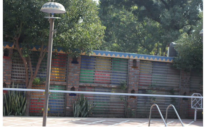
Fig. 14: Coloured cement Jalis on the boundary wall of the building of Chateau Garli, Garli, H.P.
